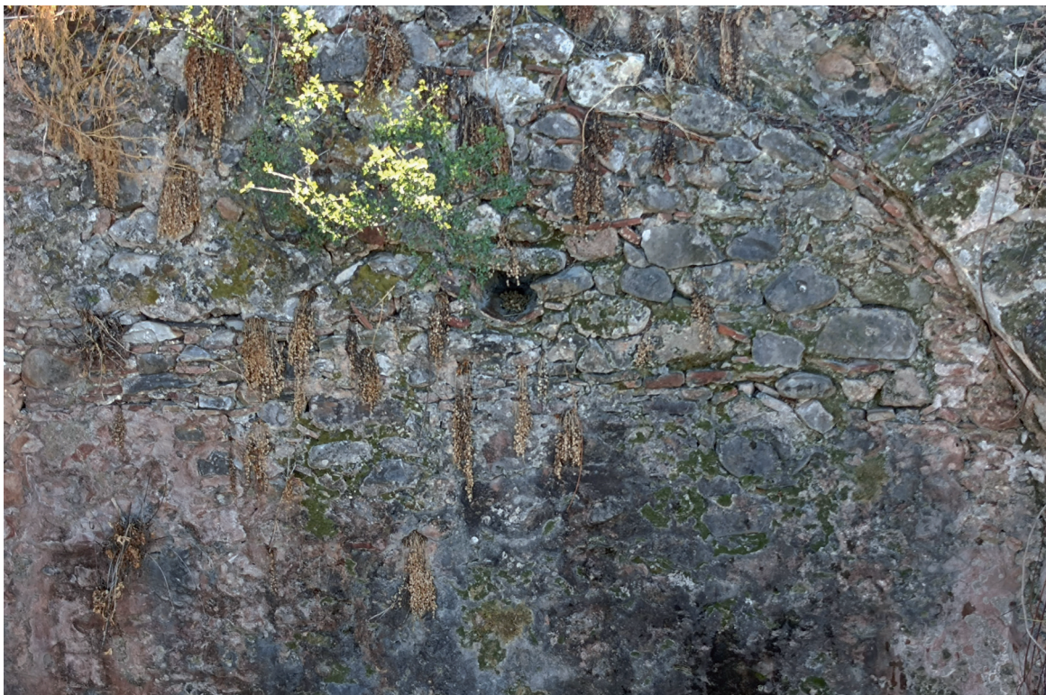
Fig. 16. Detail of the immured clay conduit at the cistern of Leuktro castle, channeling the water in the interior
