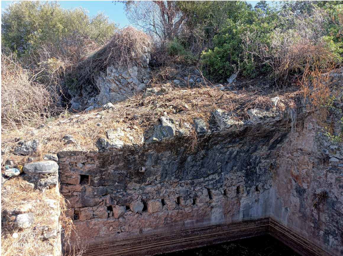
Fig. 15. The spring of the collapsed barrel vault and the beam sockets' traces of the Frankish cistern at the castle of Leuktro, in Stoupa
